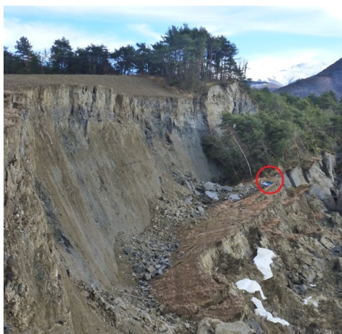
29/01/2017, the Harmalière landslide pushed away some geophysical equipment (in the red circle) ; the scarp is 10 to 15m high © Mickael Langlais
