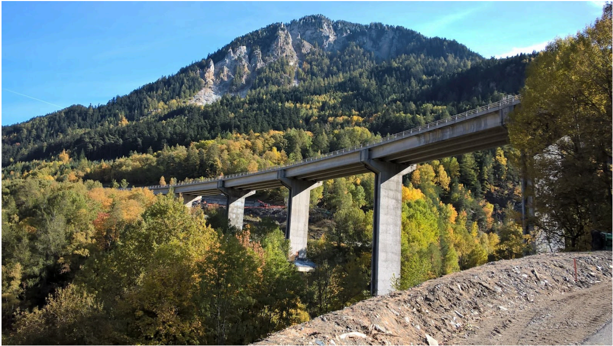
View of the ancient viaduct that will be deconstructed at ended term
