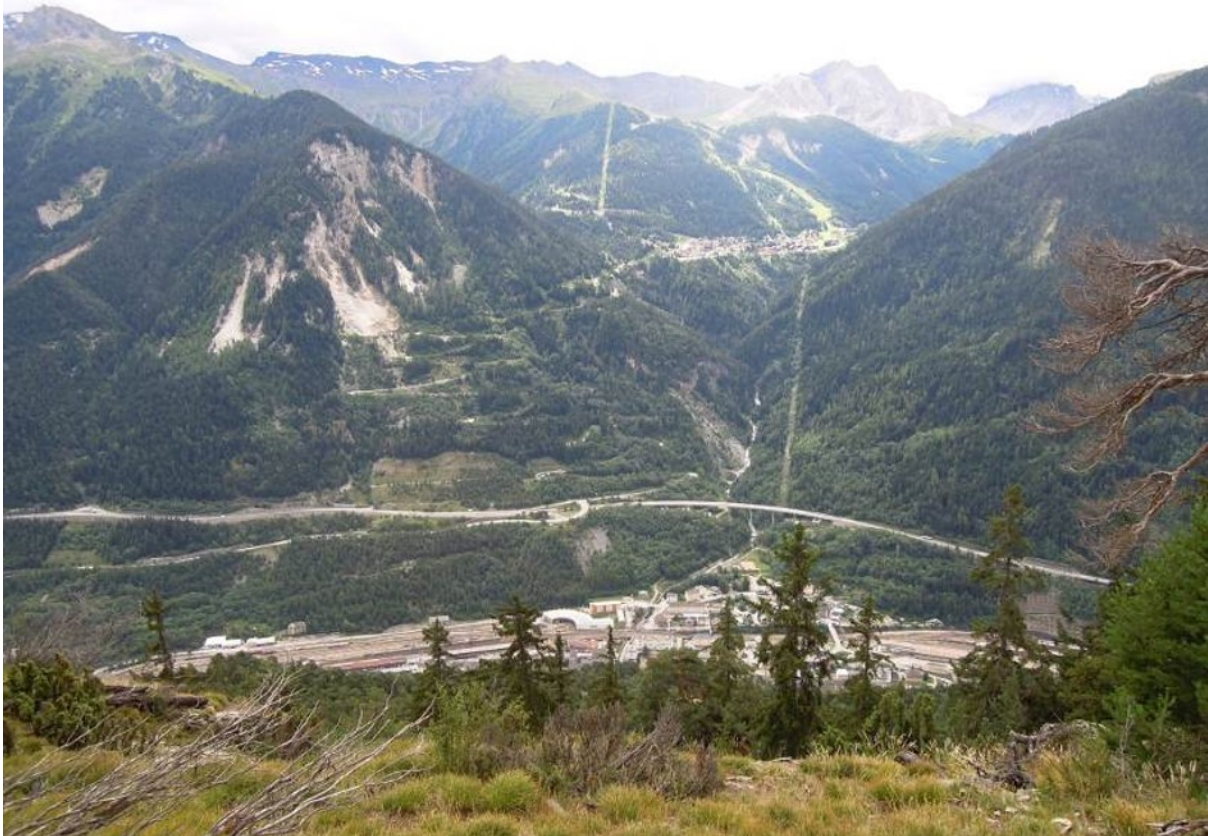
View of the Charmaix side, the access road to the head of the Fréjus tunnel and the ancient viaduct.
