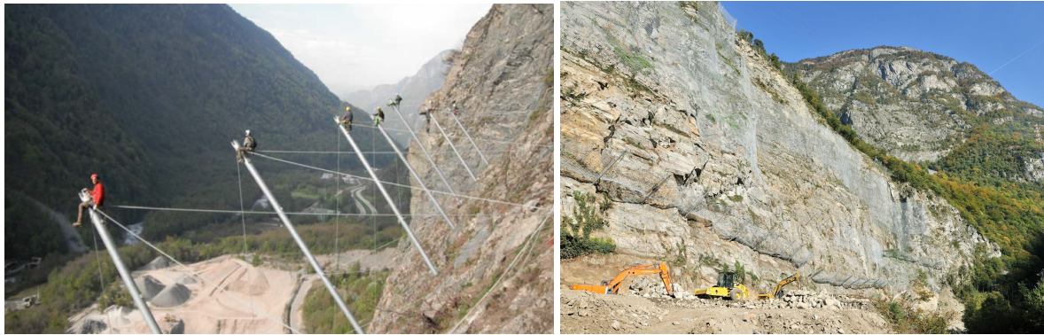
Protection works on the cliff above Romanche hydropower plant
