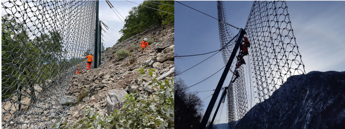
Net screens 8000 kJ - Ponsérand slope
